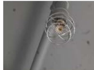
Because of the low ceilings, fire sprinklers are protectively caged.
