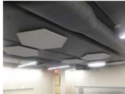
Acoustical ceiling tiles not only dampen noise, but provide a modern, decorative cover over the duct work.
