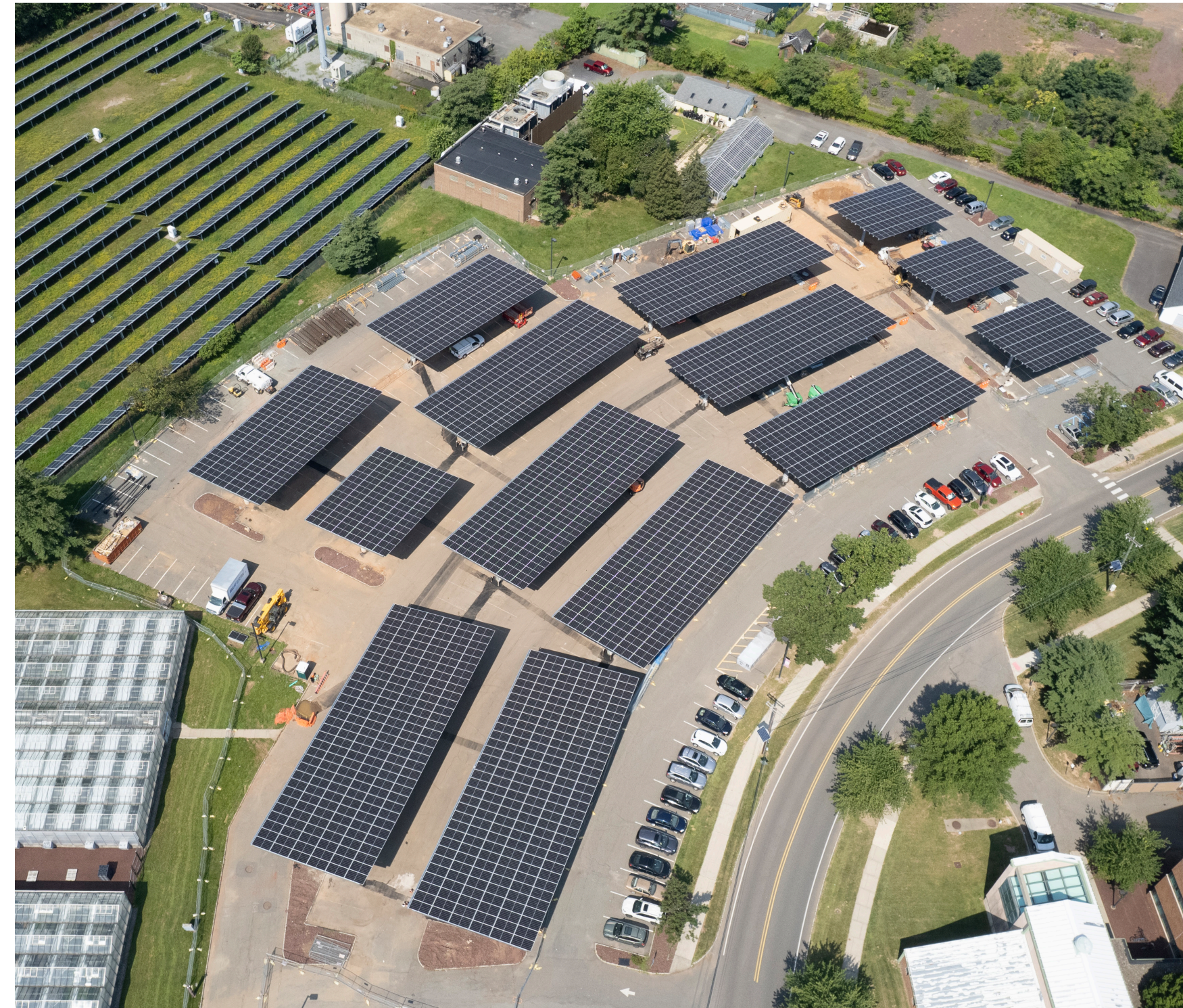
The solar canopy project neared completion in FY23.
