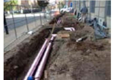
Pipe repairs on the Newark Campus.
